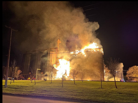
St Jean Elevator Fire—Mutual Aid
