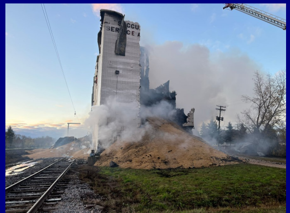
St Jean Elevator fire—Mutual Aid
